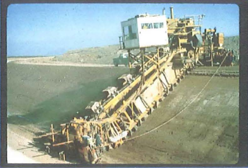
Paving The Aqueduct
