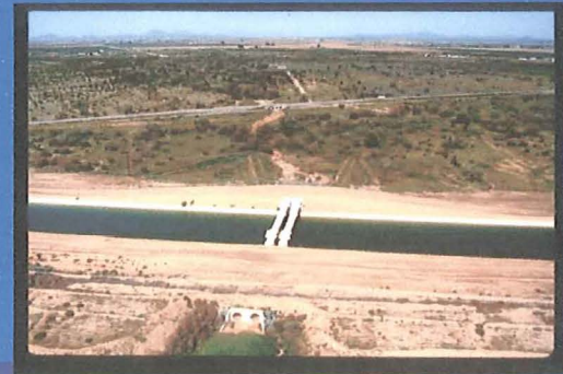
Pipe Overchute for Drainage
